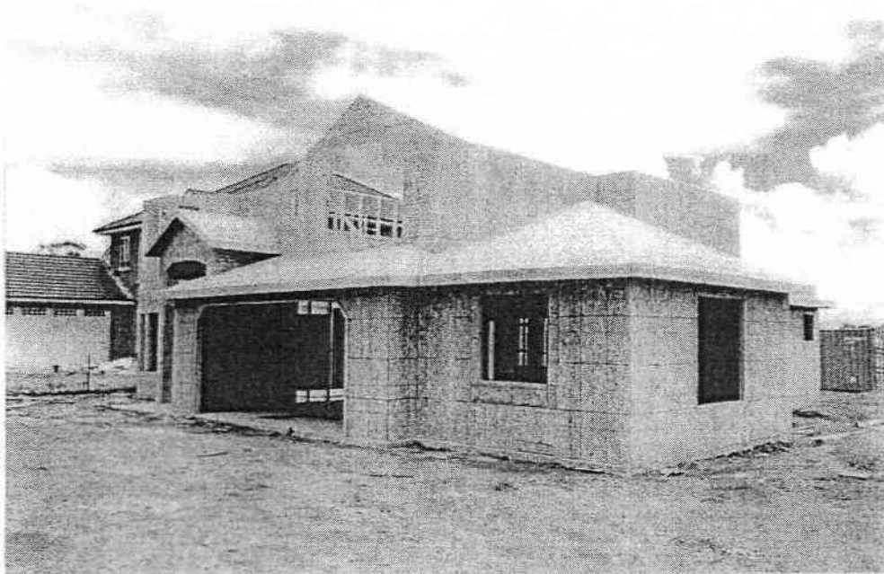
No.1 Orientated strand board - under construction.
